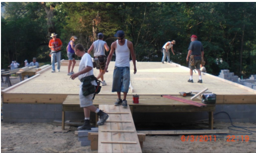
7:00am—Just a foundation and a lot of work ahead!
